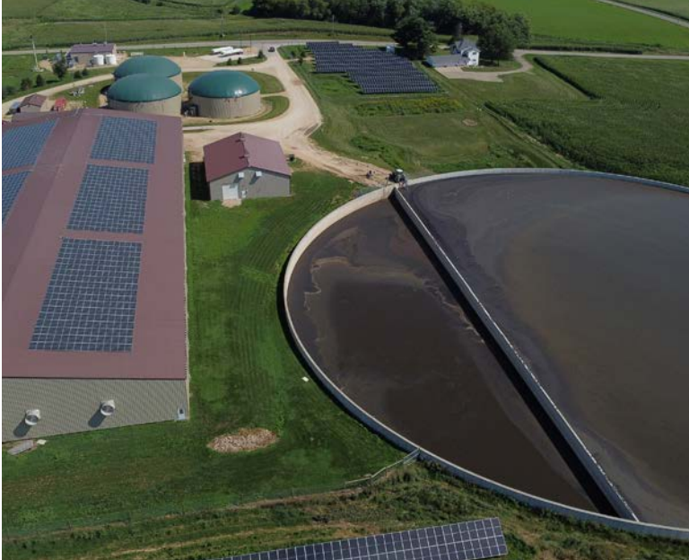
Manure digester facility in Middleton - anaerobic digester tanks, solar panels, manure storage, Solids Processing Building, Nutrient Concentration Building, and RNG Processing Building are visible
