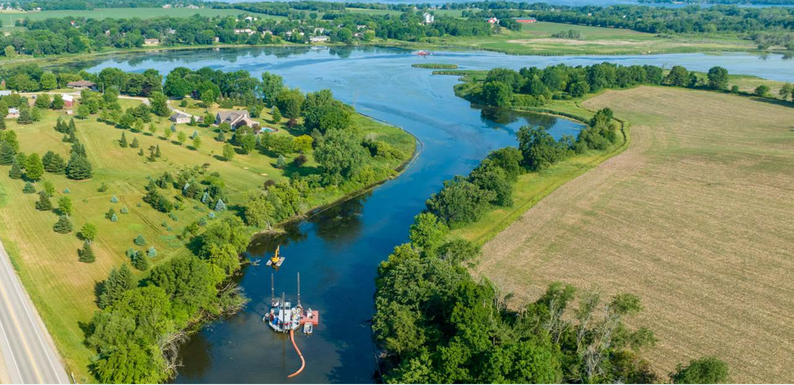
Yahara River sediment removal southeast of Lake Kegonsa near County Highway B. This is Phase II of a five-phase plan that will help reduce flooding for all lakes once completed in 2026. Photo courtesy Robert Bertera.
