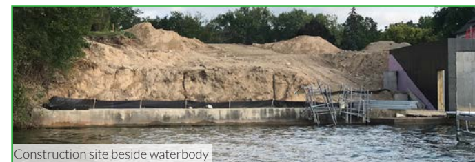
Construction site beside waterbody
