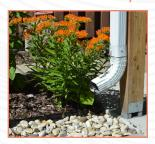
This simple action allows you to redirect rainwater to your lawn or garden, while also reducing the amount of stormwater that goes to streets and directly into the lakes via storm sewers.
